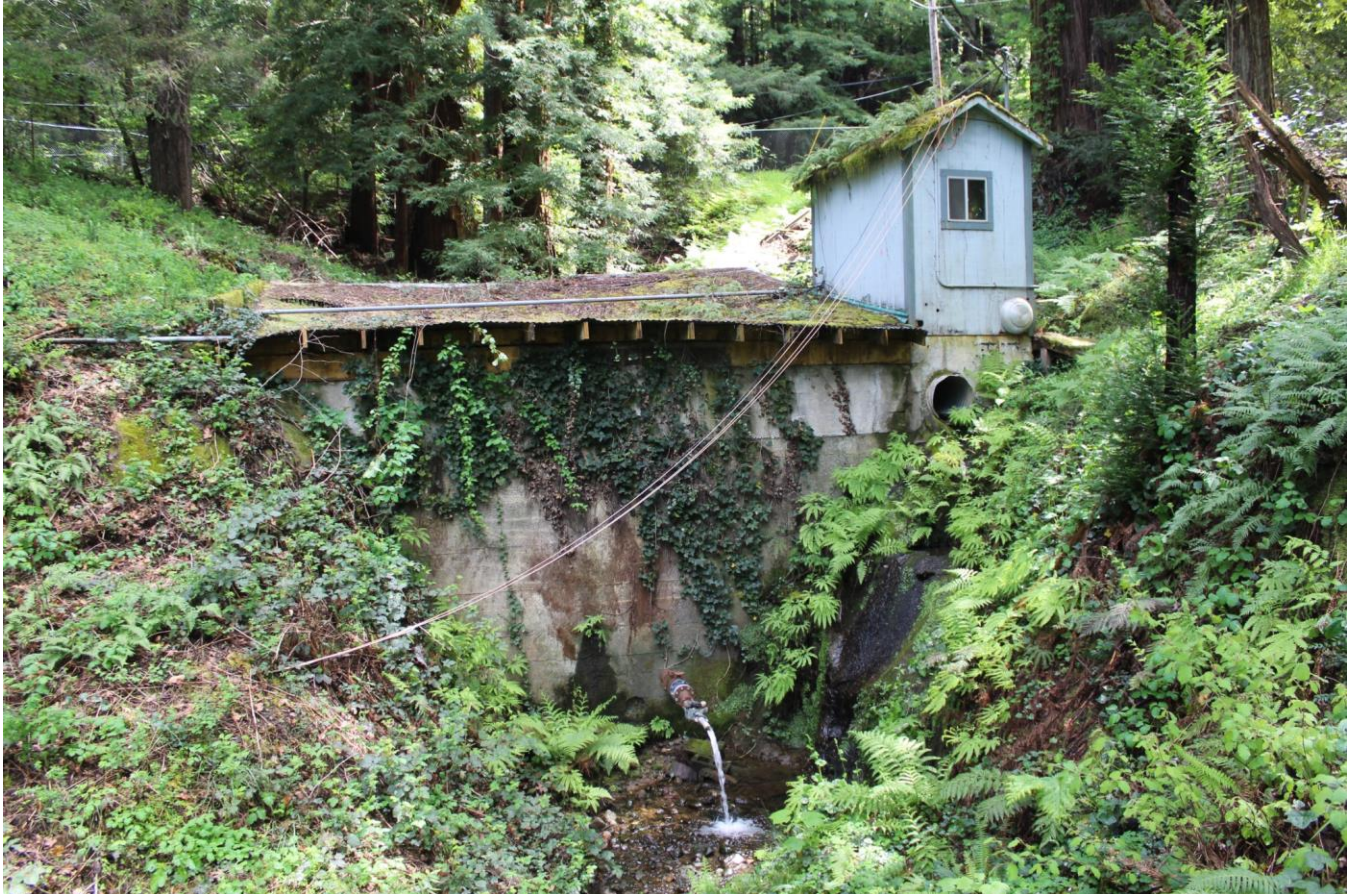
Existing spring structure spanning the drainage ravine at the project site.
