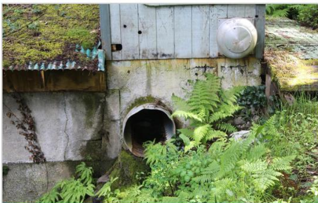
Outlet / structure base condition
