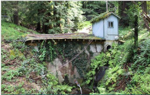
Structure overview across drainage
