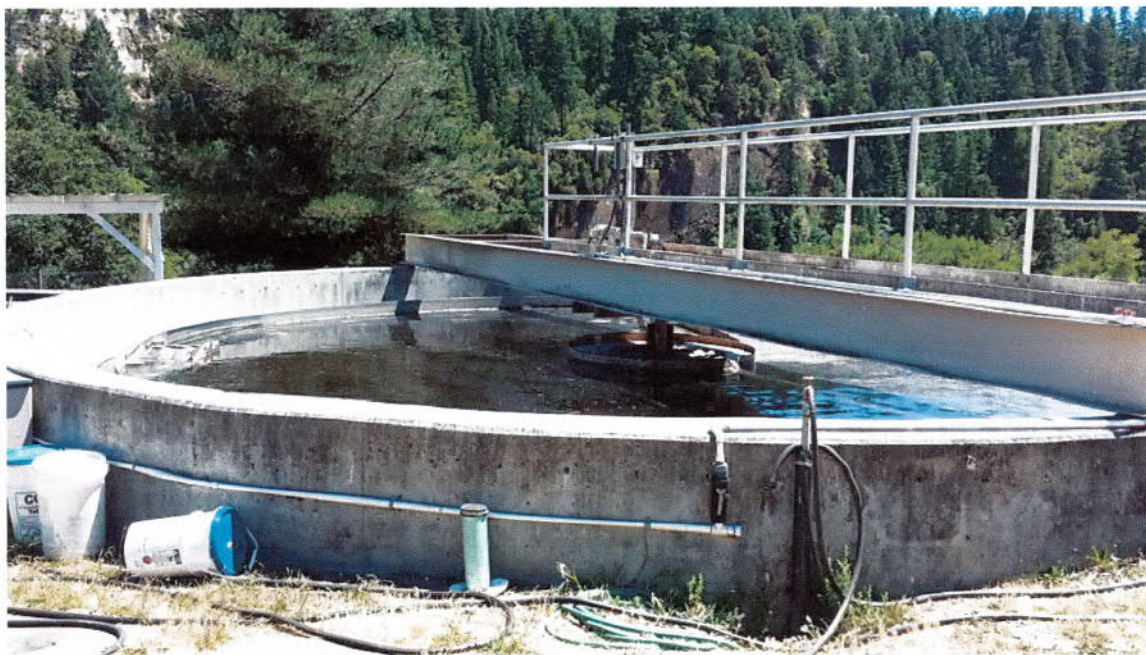
Figure 11. 36 Foot Diameter Secondary Clarifier
