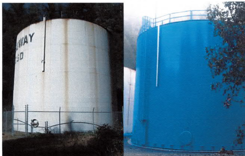
Figure 5. The New 460,000 gallon and Original 275,000 gallon Rusk Avenue Tanks.
