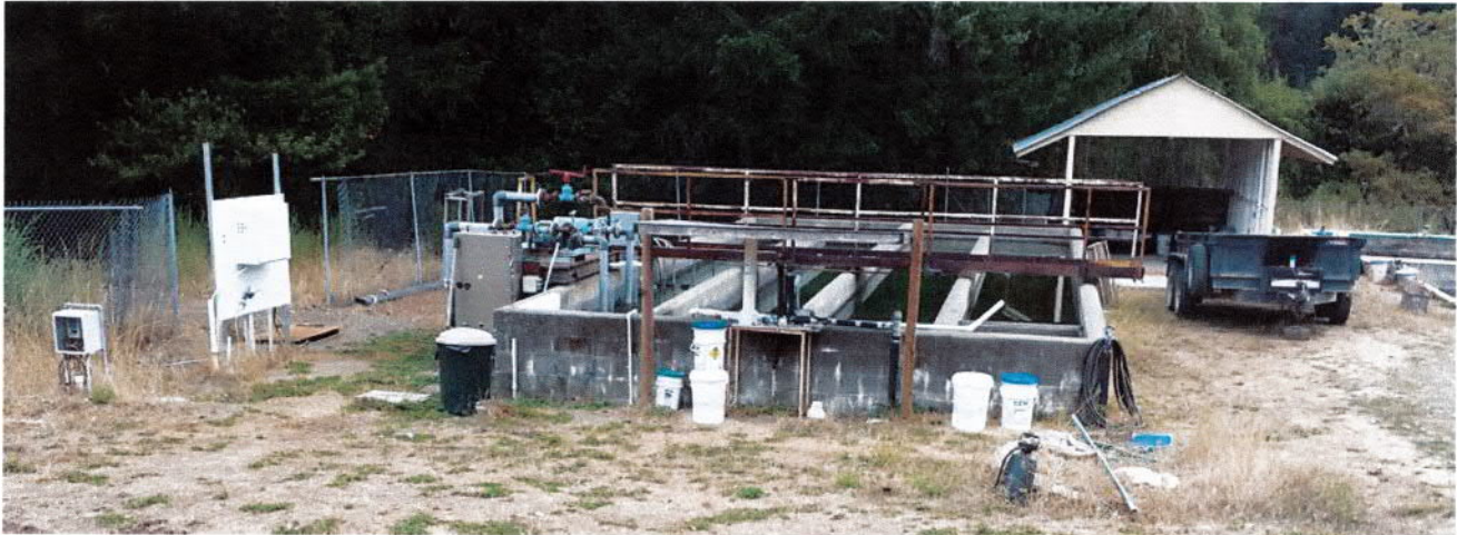
Figure 13. RCSD WWTP Chlorine Contact Basin
