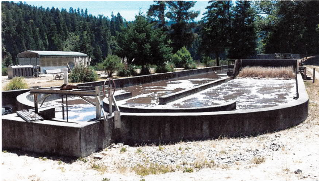
Figure 10. 300,000 Gallon Single Loop Oxidation Ditch
