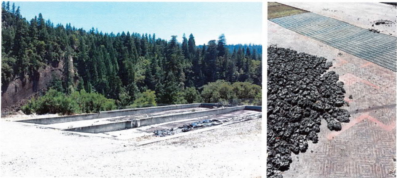
Figure 14. Sludge Drying Beds and Drainage Tiles
